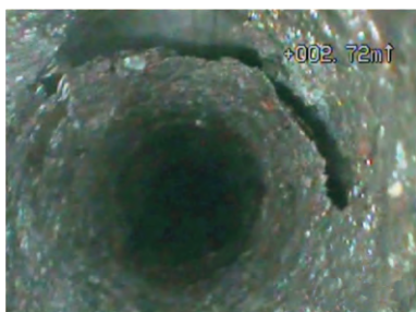
Fig. 2 - Heavy corrosion inside a cast iron downpipe.
