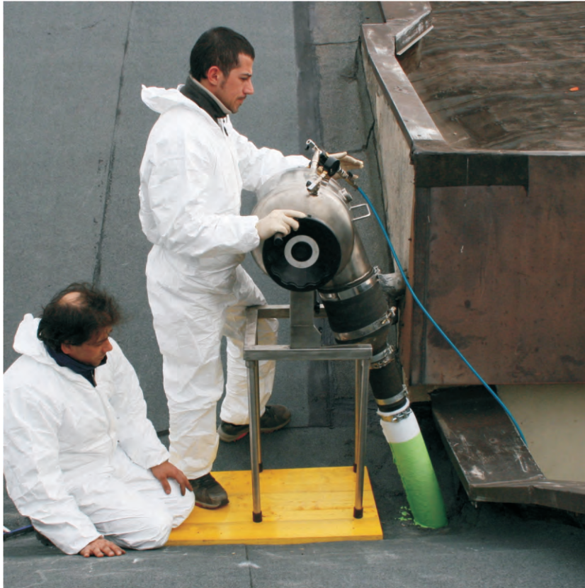
Fig. 8 - The liner is inverted inside the pipe to be repaired. In this way the resin is on the outside of the liner, in direct contact with the walls of the pipe.
