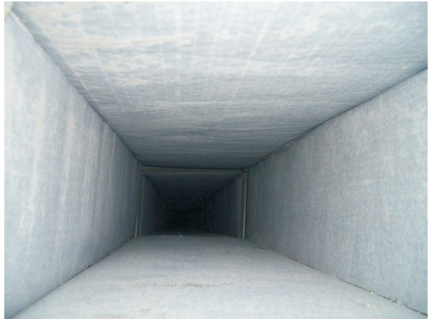
Fig. 16 - An air-conditioning duct after treatment with anti-bacteria long term sanitization process .
