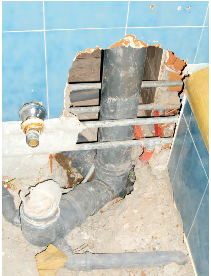
Fig. 5 - repair of a Y-branch carried out using traditional techniques, involving the usual and unwanted demolition (Photo by Renato D'Apuzzo).
