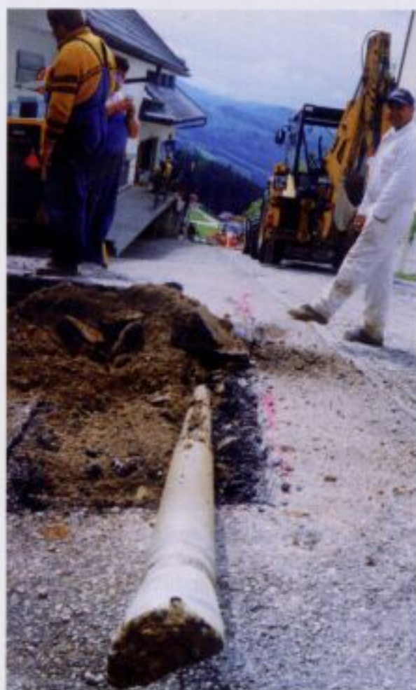
The Scorpio DDD drill head emerging after completing a pilot bore.
