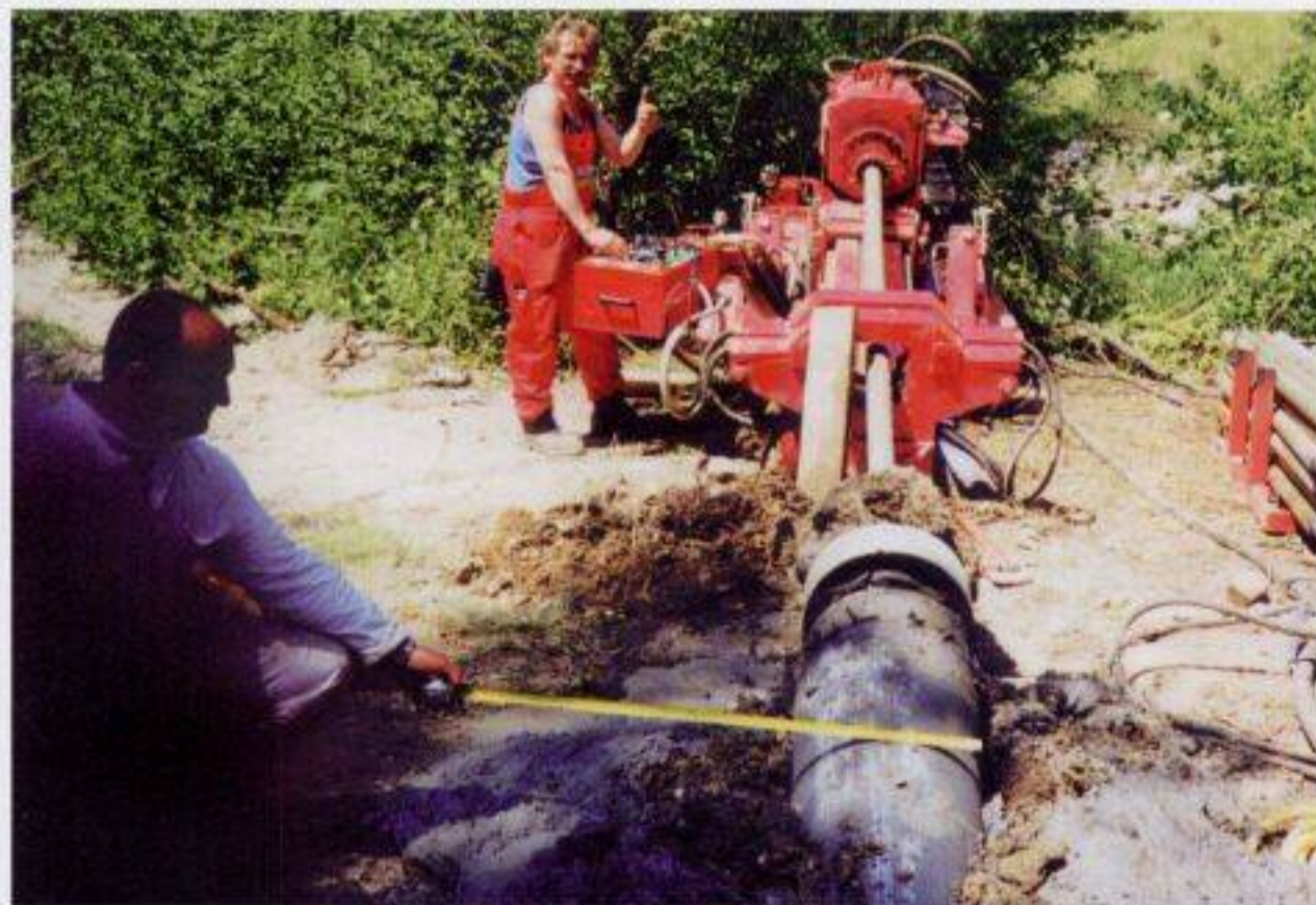
A Scorpio drill rig completing a pipeline pullback operation.
