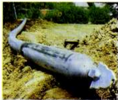
FIG. 8 - Pipe splitting
